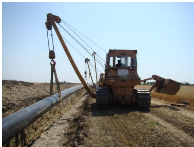
Figure 2: Laying a section of pipeline into the trench
