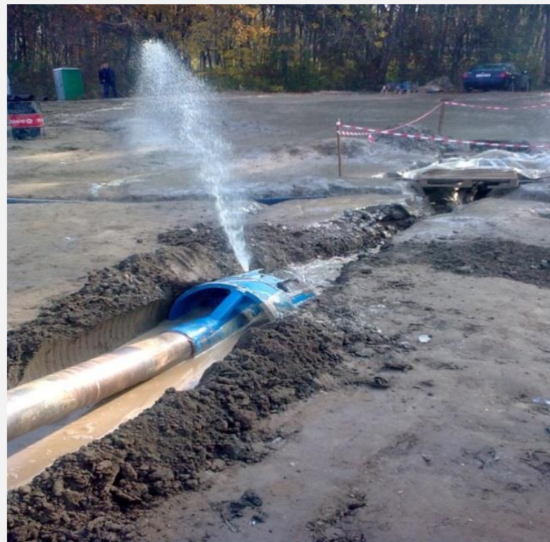
Drilling bit (500 enlarger) – drilling works to tow the main pipeline
