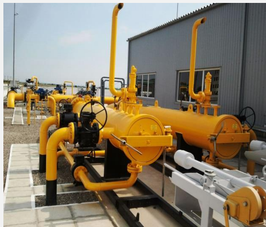
PIG launching/receiving trap
