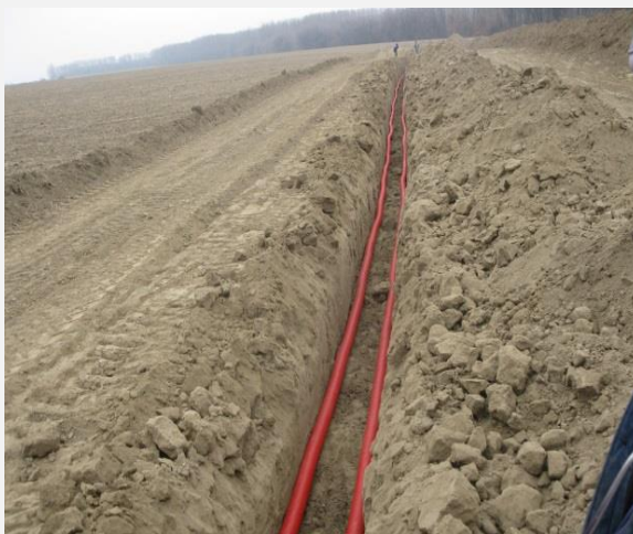
Fiber optics towed in protection pipe
