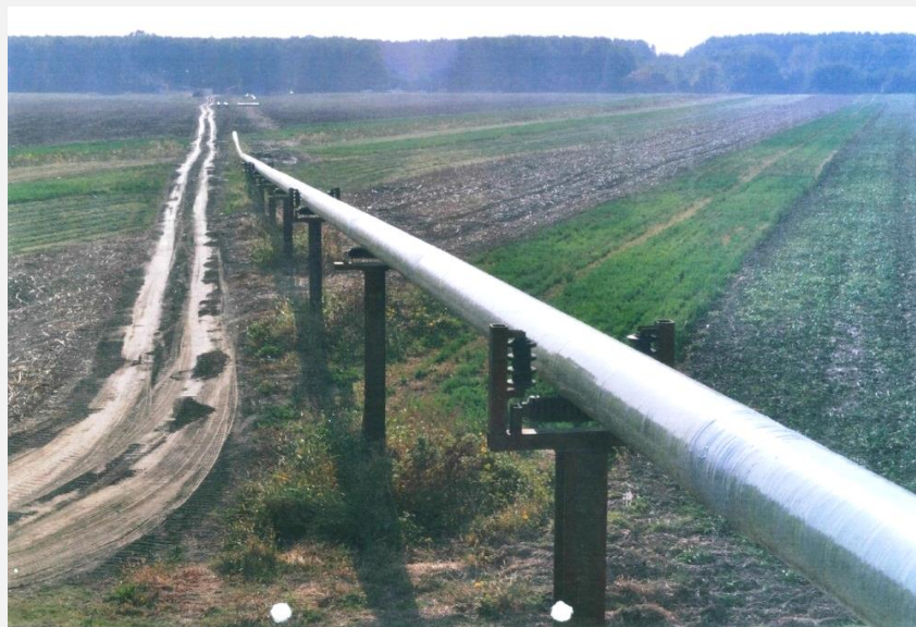
The main pipeline on the Romanian territory – prepared to be pulled into the Danube bottom
