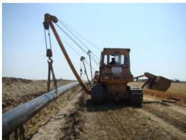
Figure 4. Laying a section of pipeline into the trench
