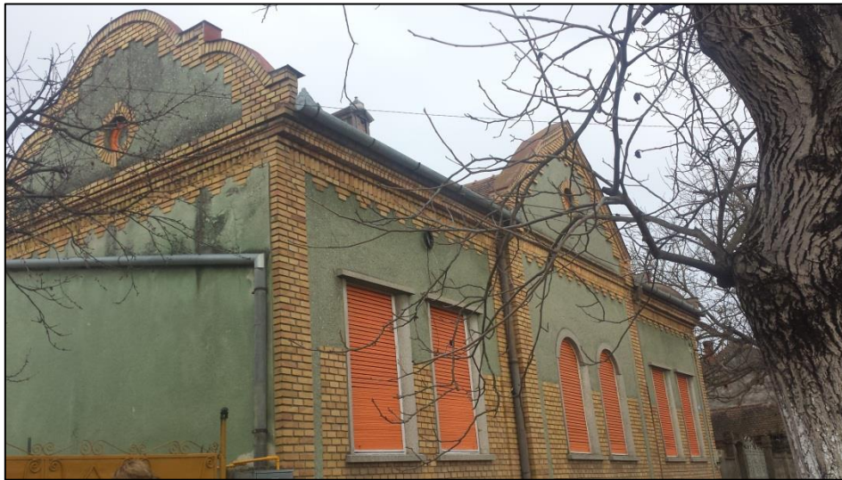
Figure 12. House in Coşteiu, Timiș County
